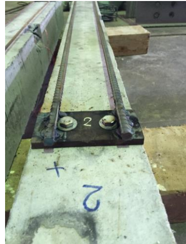
Figure 6. Welding of steel bars with steel plate
