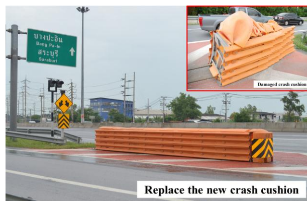
Figure 14. The replacement of damaged devices
