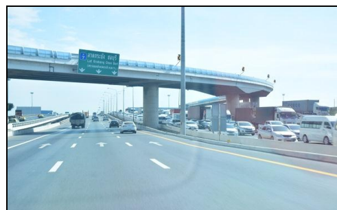
Figure 5. Problems on roadside hazards: height of concrete barrier
