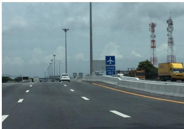
Figure 15. Raising of concrete barrier height
