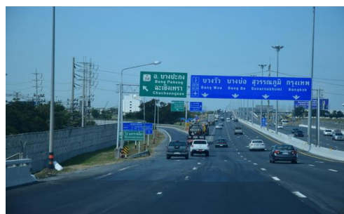
Figure 4. Problems on alignment, roadside hazards, markings and pavement
