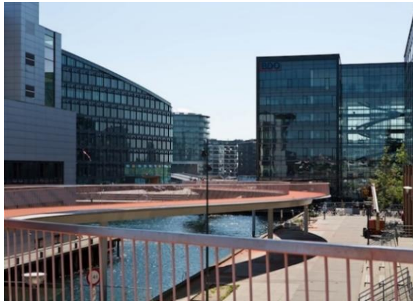
Figure 7 “Cykelsangen” (Bicycle Snake Bridge) in Copenhagen [18]
