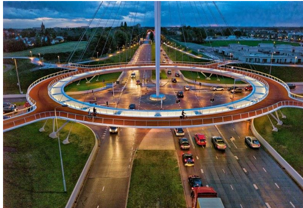
Figure 6 “Hovenring” in the Netherlands [17]
