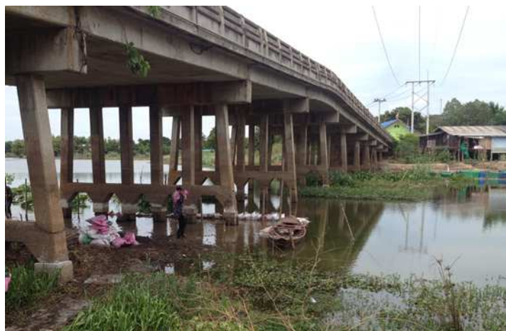
Figure 1. Photograph of bridge and site condition
