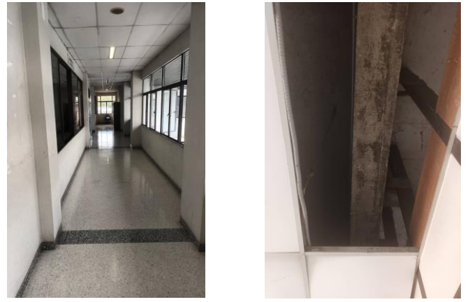
a) Floor and windows Fig. 1 Laboratory building
