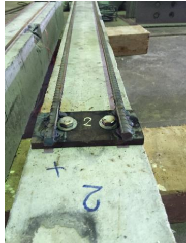
Figure 6. Welding of steel bars with steel plate
